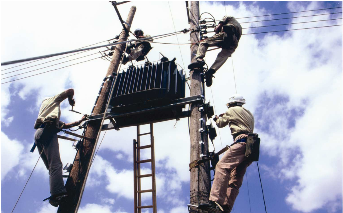
Photo Installation of overhead transformer of the EAC
